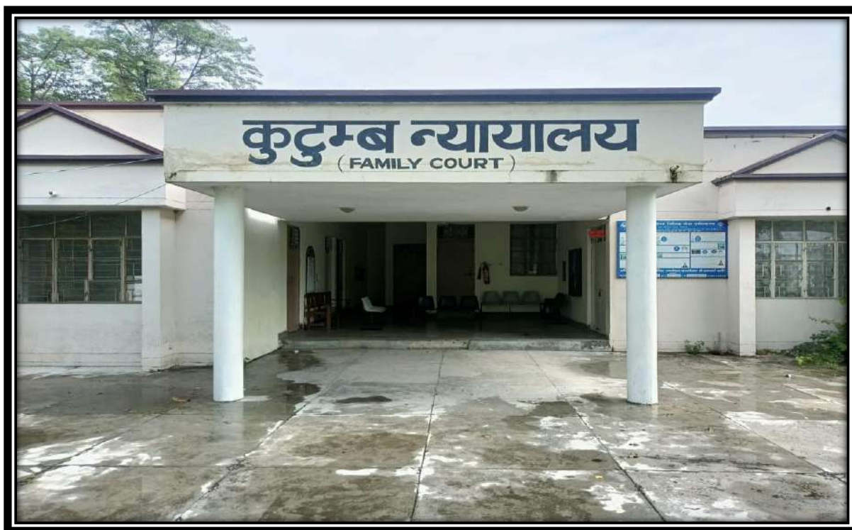
Family Court I Building, Rudrapur, U.S. Nagar
